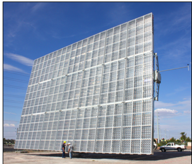
Figure 3.7 Amonix Solar Concentrating PV Module. Source: Amonix Solar http://www.amonix.com/products/index.html .
